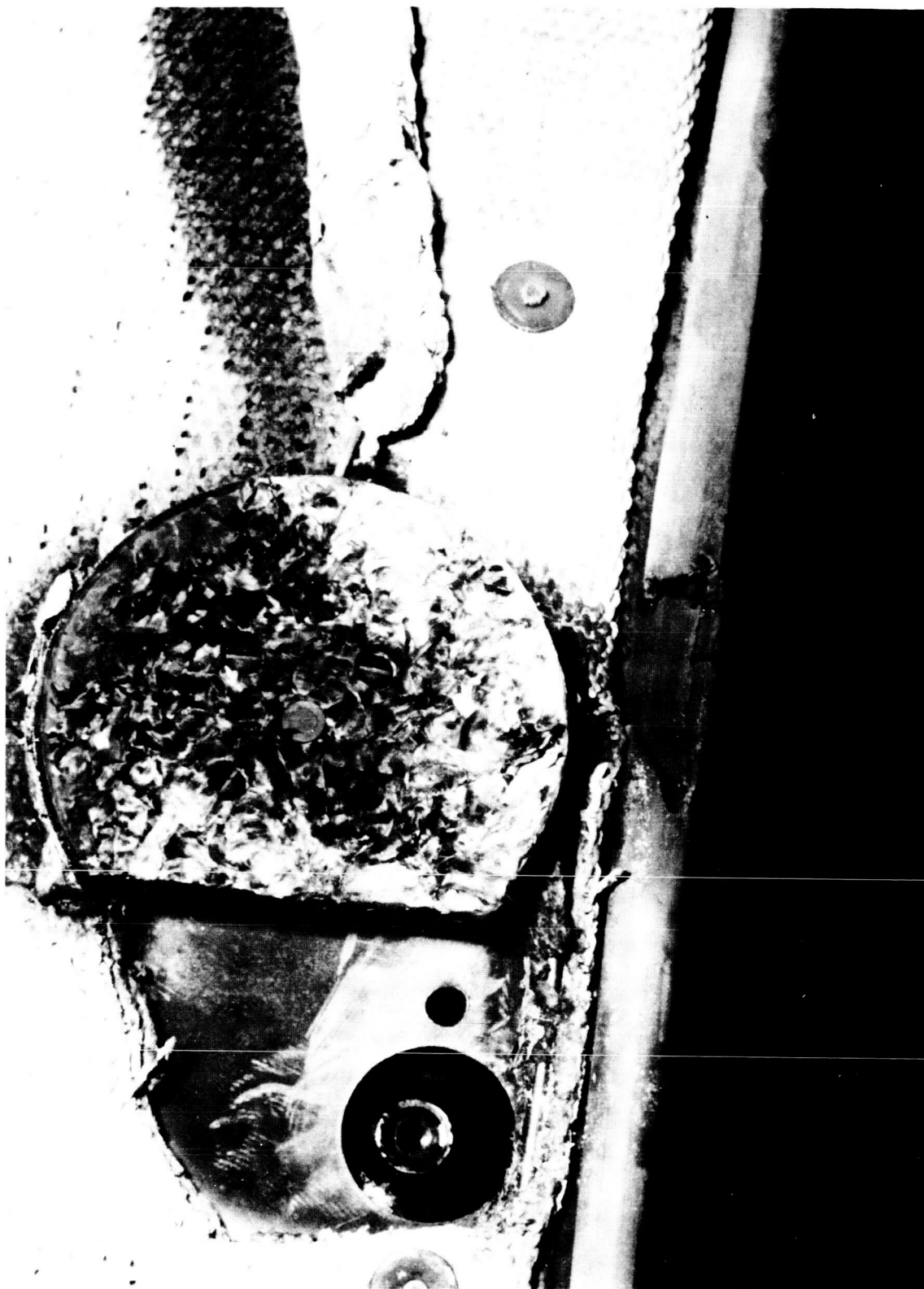
FIGURE 2-4 METAL EROSION, ASPIRATOR LIP OF ENGINE 3
