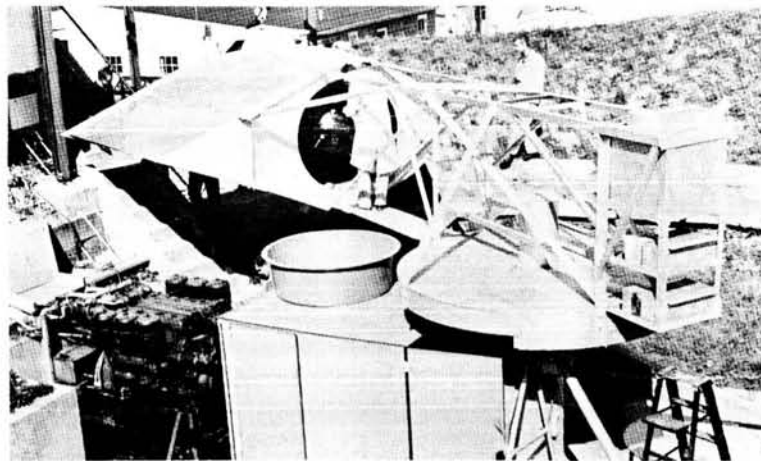
Figure 3.—Prototype spacecraft installed on centrifuge for acceleration.
