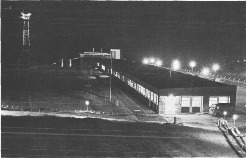
Fig. 8—View of the main building at night.
