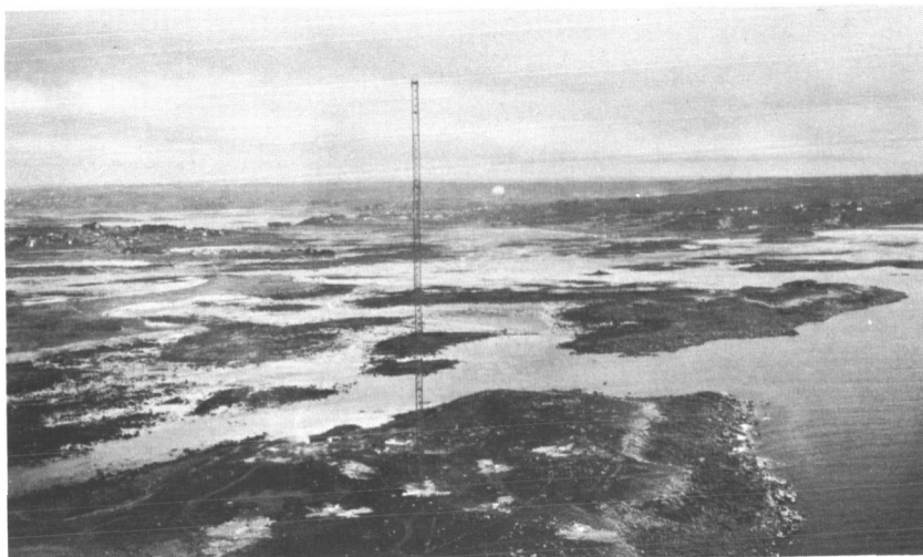
Fig. 12 — View of the Ile Losquet and the 200 m tower.
