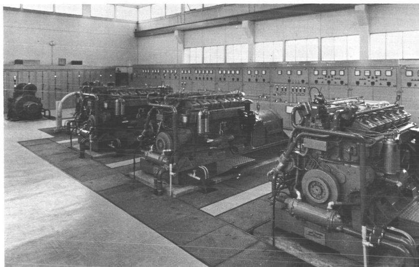
Fig. 37 — Interior view of the power supply building.
