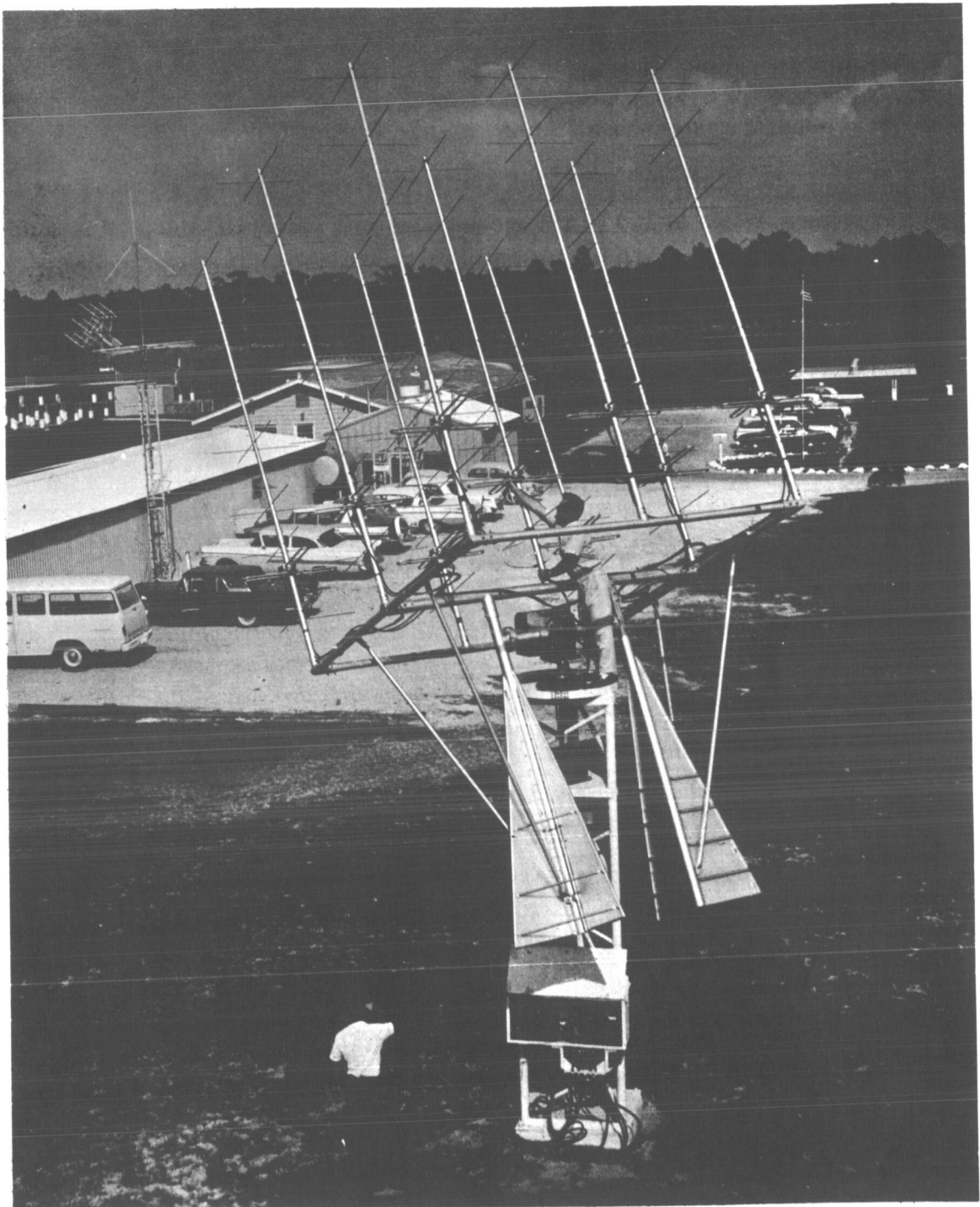
Figure 11. A 9-Yagi, 136-Mc STADAN antenna.
