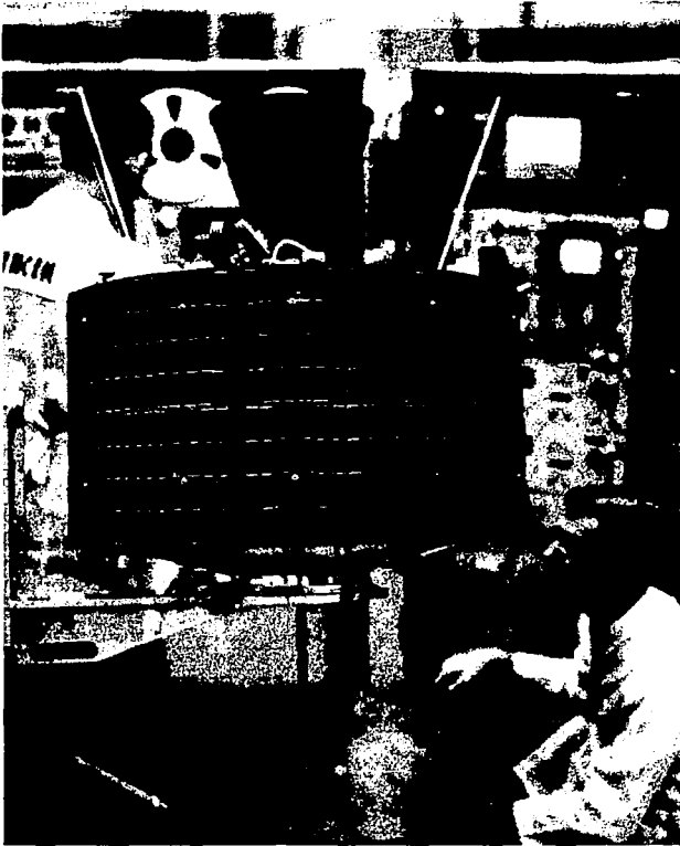
Figure II-2—Syncom C, side view with solar panels.
