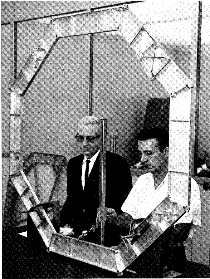
Fig. 9. Primary structure lower ring
