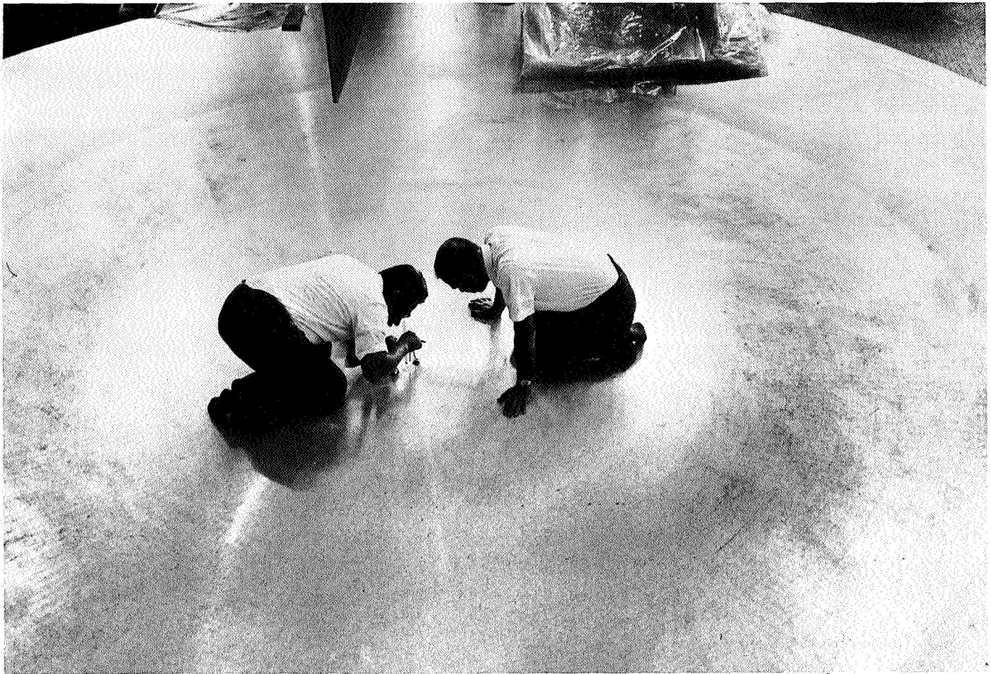
Fig. 2. Locating center of mirror
