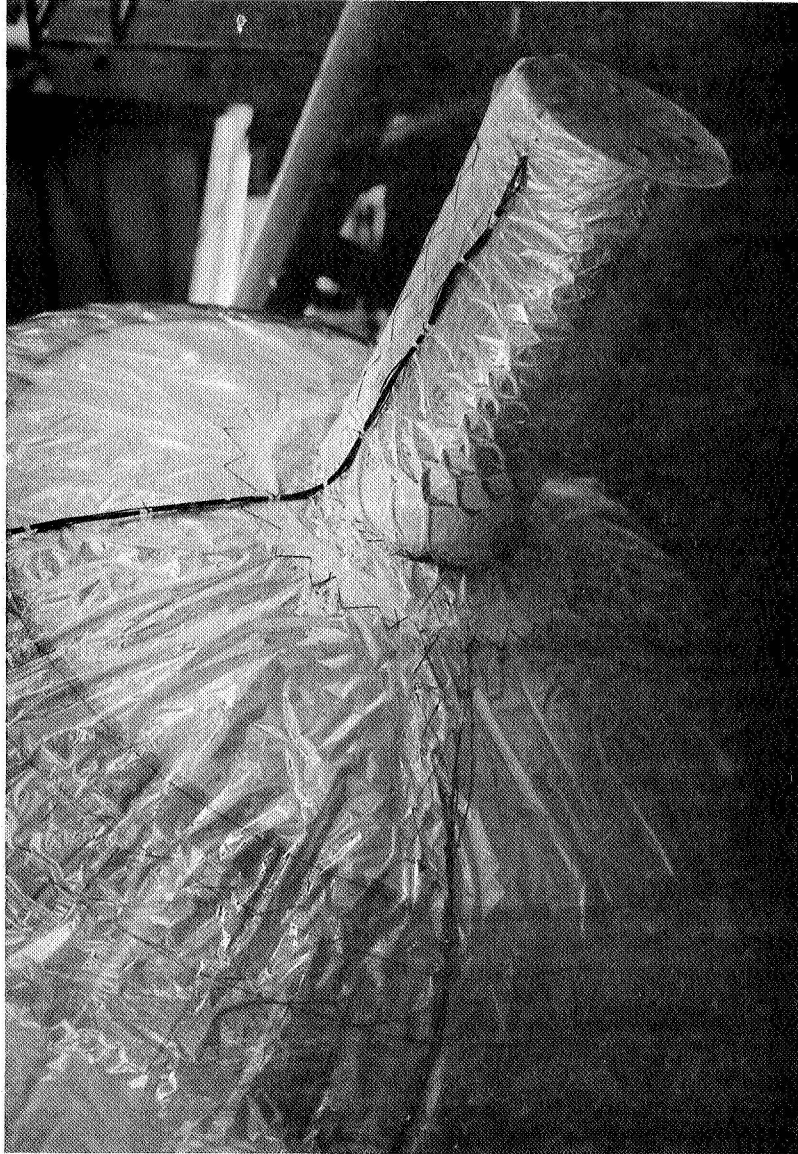
FIGURE 28 INSULATED "A" CAP PIPE PENETRATION
