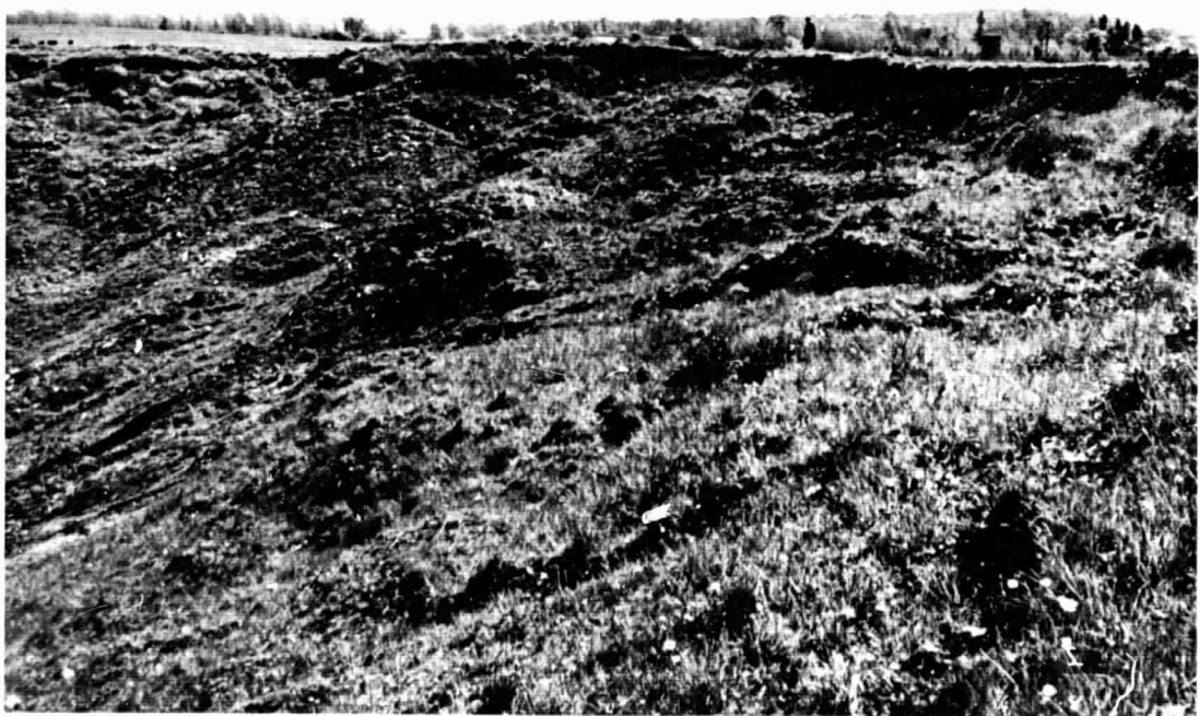
Fig. 6 Ground-based photograph taken in 1967 showing slumping of materials forming inner rim of Fauld crater.
