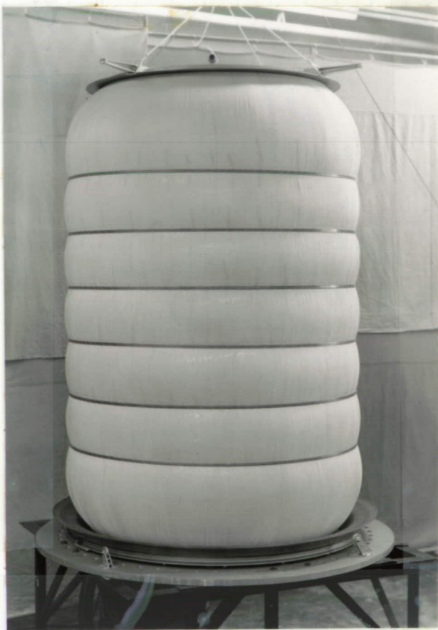
Figure 23. Pressurized Structure Ready for Installation of Micrometeoroid Foam and Dacron Fabric
