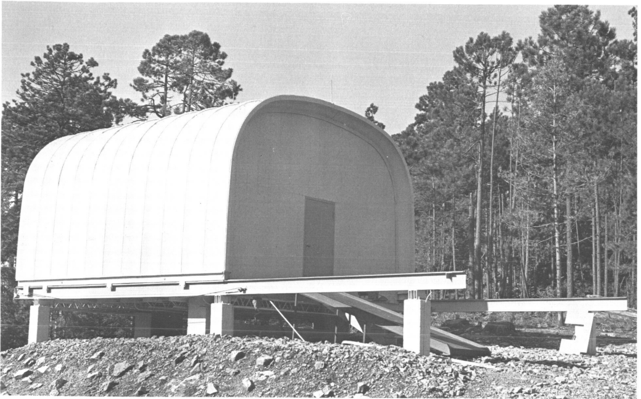
Fig. 2 The roll-off-roof building which houses the 28-inch telescope. The south wall of the building (at left) is hinged and folds down for observations of southern stars.
