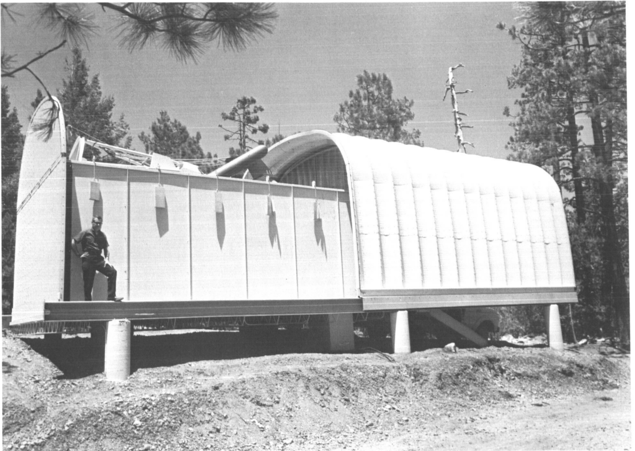
Fig. 8 The roll-off-roof building which houses the 60-inch photometric telescope. The telescope is shown in its rest position. The south wall of the building (at left) is hinged and folds down for observations of southern stars. The hanging weights counterbalance the wind screens.
