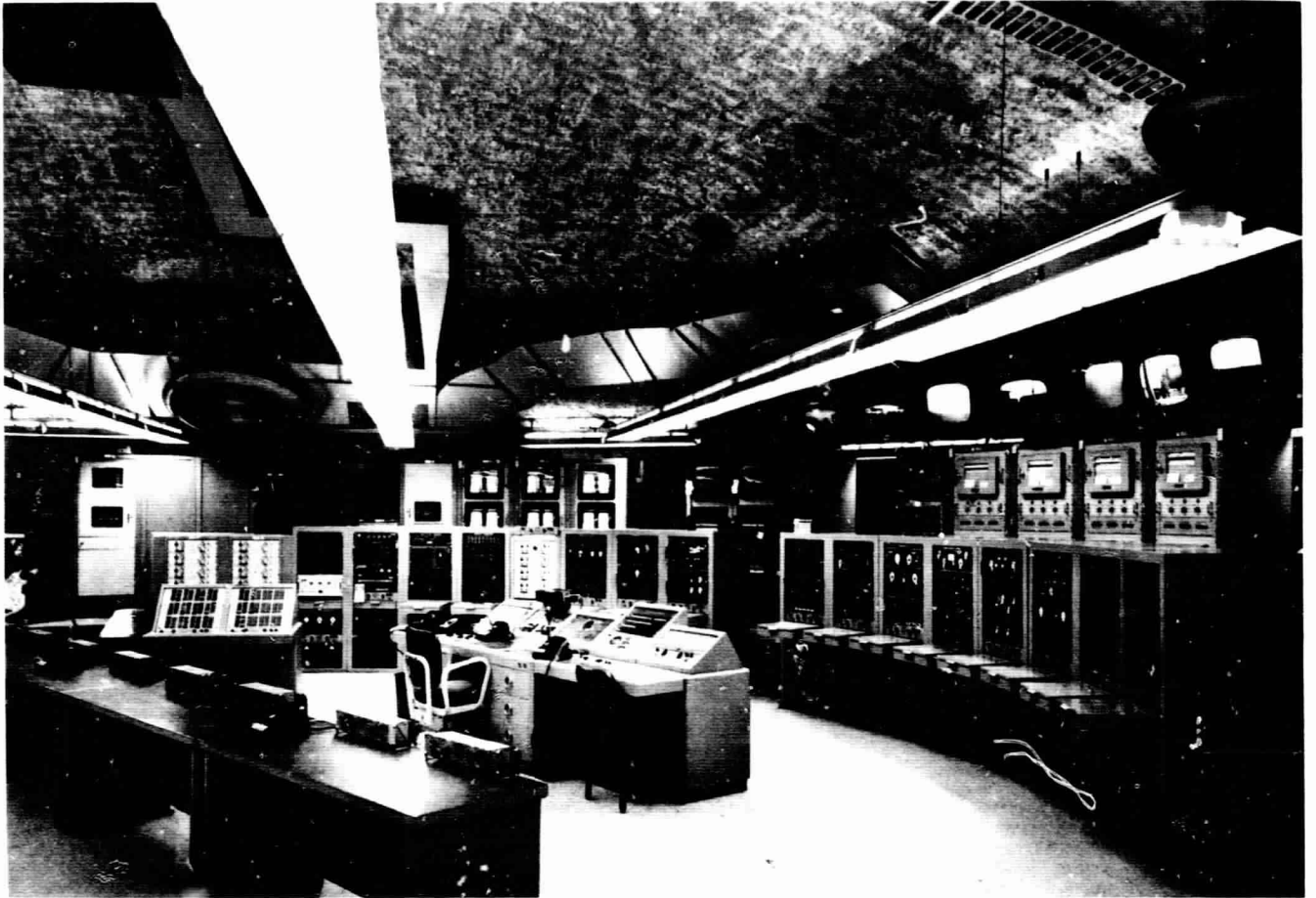
Fig. 4. Launch complex blockhouse
