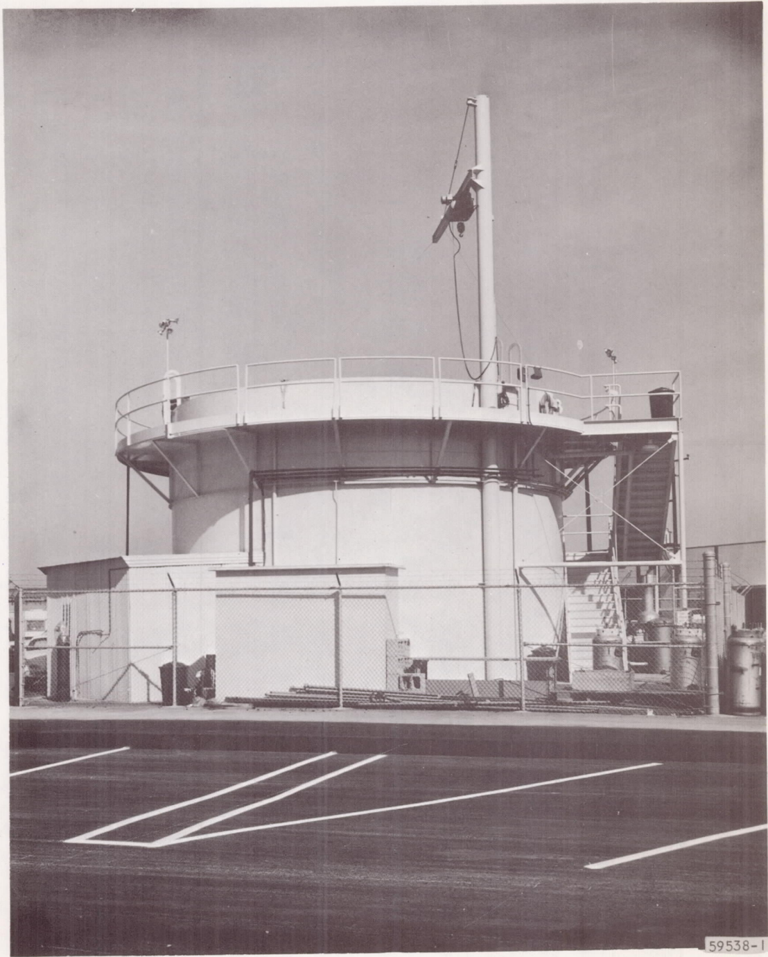
Figure 2-1. Underwater Test Facility
