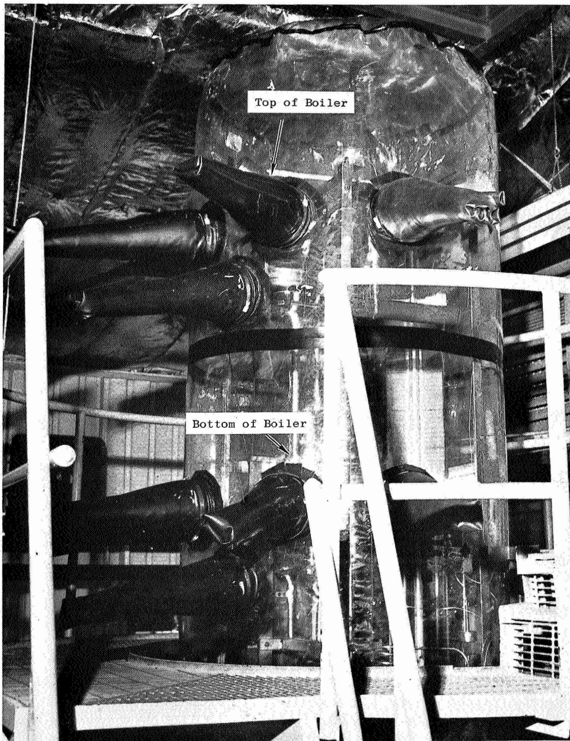
Figure 6. Vinyl Chamber Used for Cutting Operations on Boiler of T-111 Corrosion Test Loop. (C68062842)
