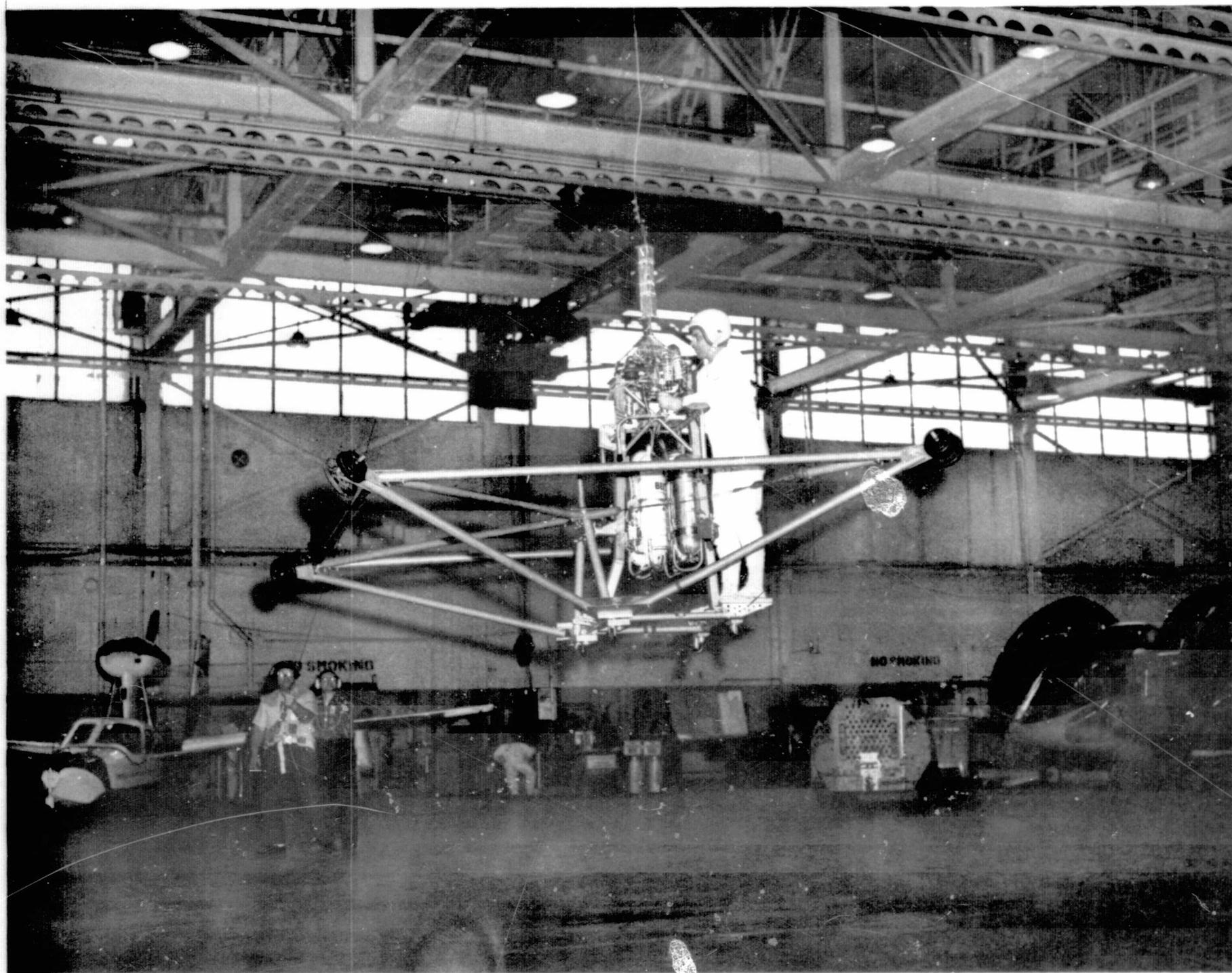
Figure 2. 1-g Kinesthetic Vehicle (High Inertia)
