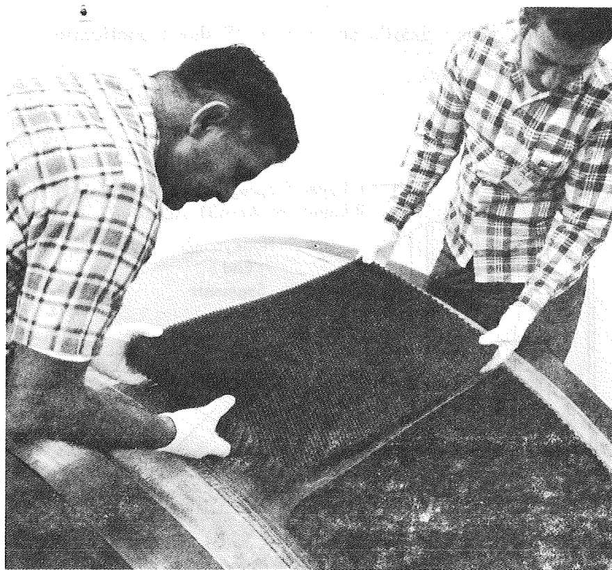
Figure 47: CORE CENTER SECTION PLACEMENT
