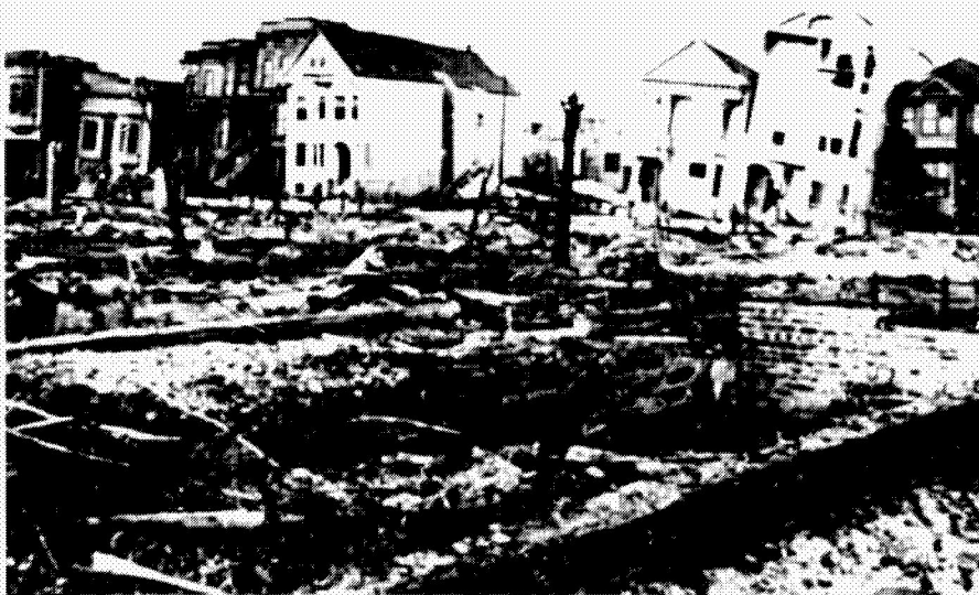
FIGURE 4 Damage to buildings on Howard Street, San Francisco, resulting from 1906 earthquake. (Photograph from University of California, Berkeley.)
