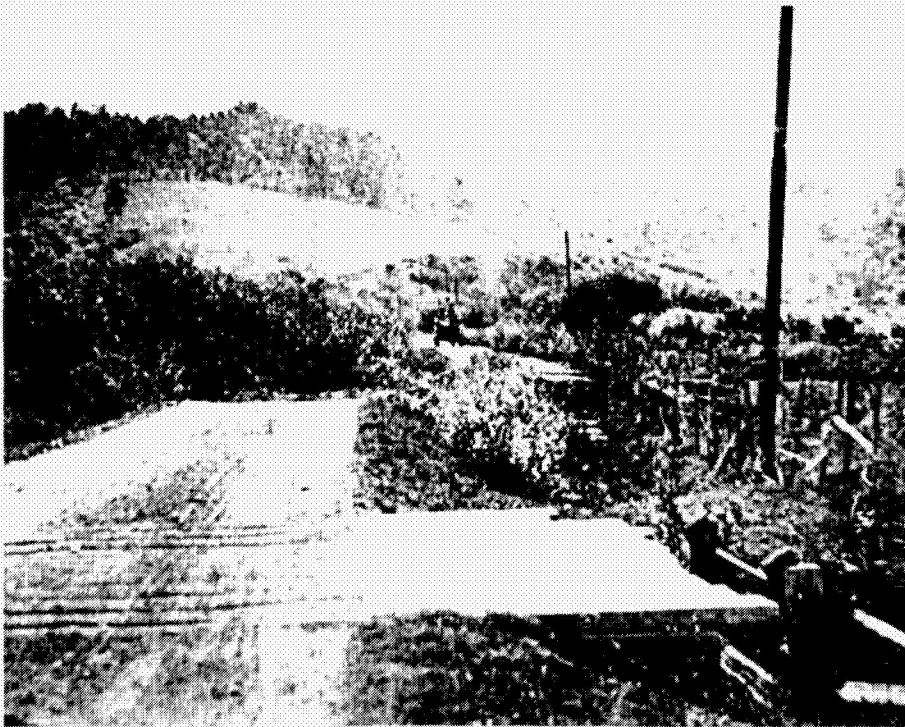
FIGURE 9 Offset of 21 feet in a road at the south end of Tamales Bay, California, resulting from the 1906 earthquake. Road segment at lower left was formerly joined to partly obscured segment in exact center. (Photograph from University of California, Berkeley.)
