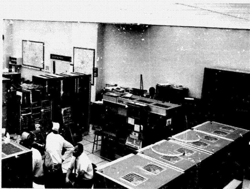
FIGURE 17 Interior of LASA Data Center at Billings, Montana, where all signals from the 525 LASA sensors are brought together for automatic processing. The Center, nearly 150 miles from the array center, serves as a research facility where scientists and engineers from many organizations can conduct independent research. (Photograph from Lincoln Laboratory, MIT.)
