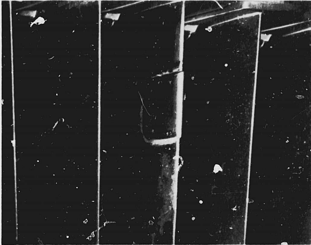
Figure 16. Wrap-around Bucket Brazed Patch
