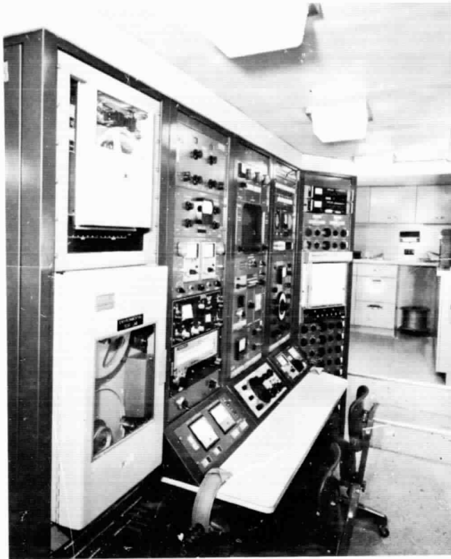
Fig. 37. Vibration control console
