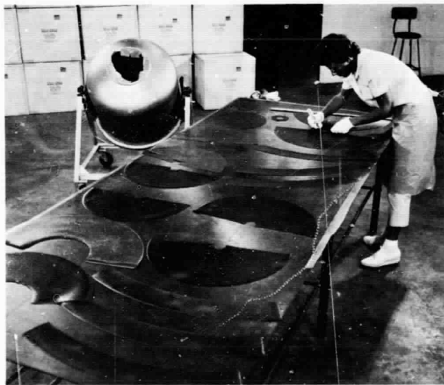
Fig. 13. Chamber insulation pattern pieces
