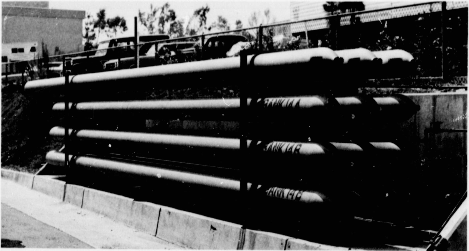
Fig. 22. Gas storage tanks
