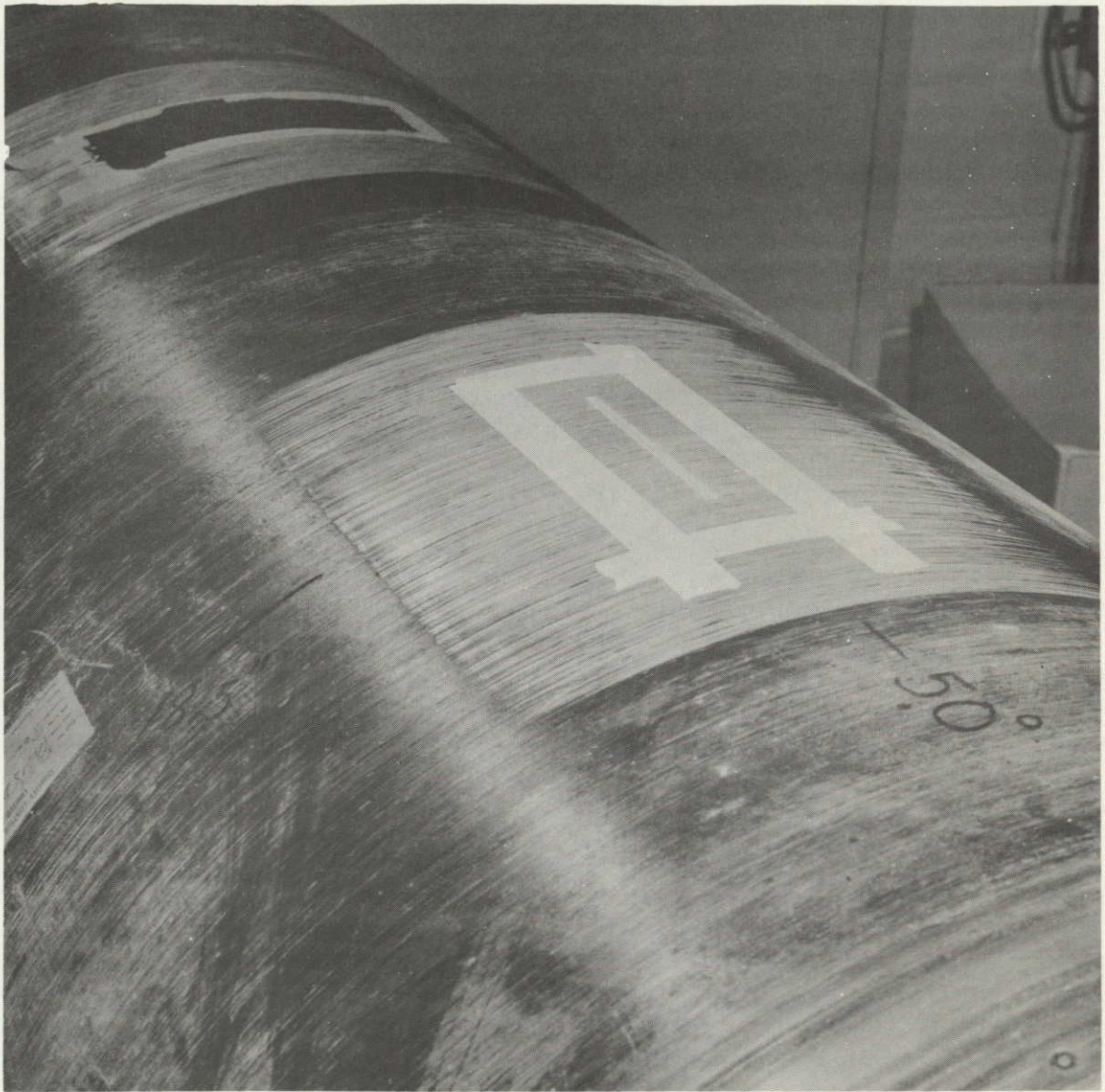
Figure 62. Repair Areas with Precoat area Marked
