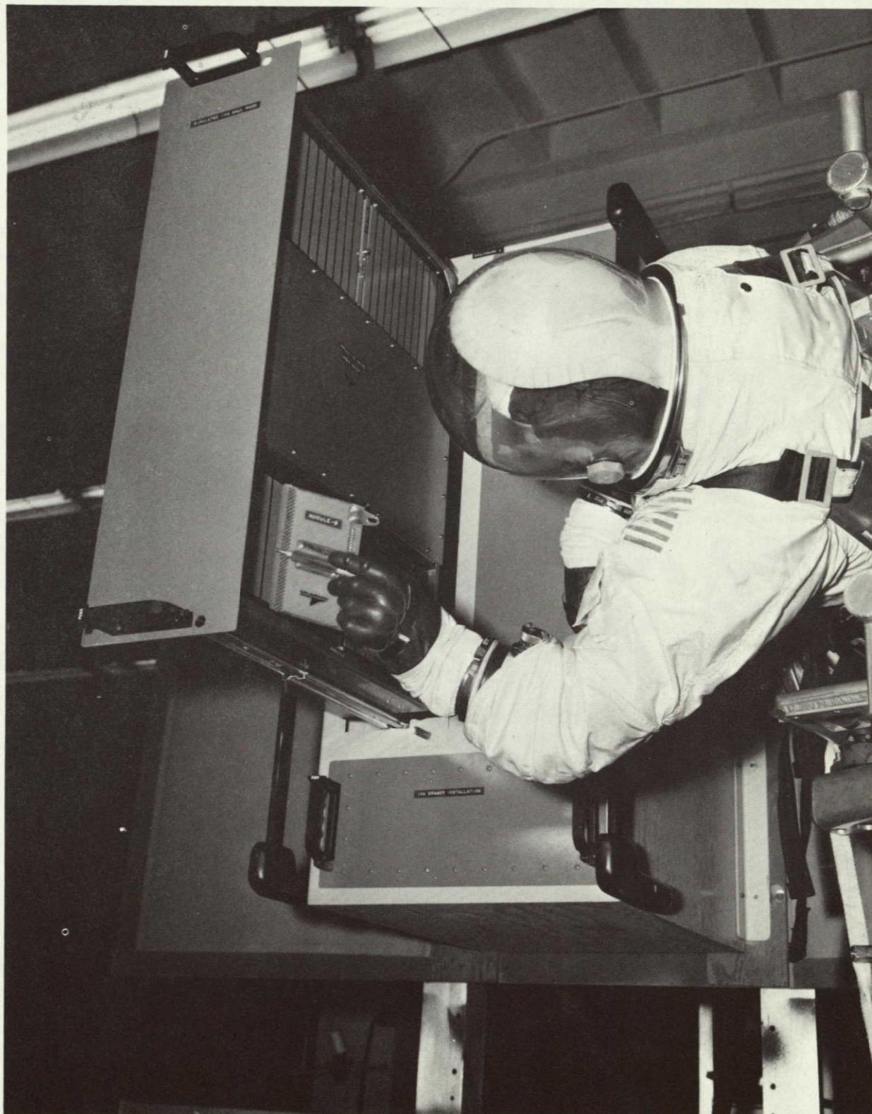
Figure 10-14. Installing IVA Module #9 Pressure Suit With IVA Gloves Zero-g Simulation
