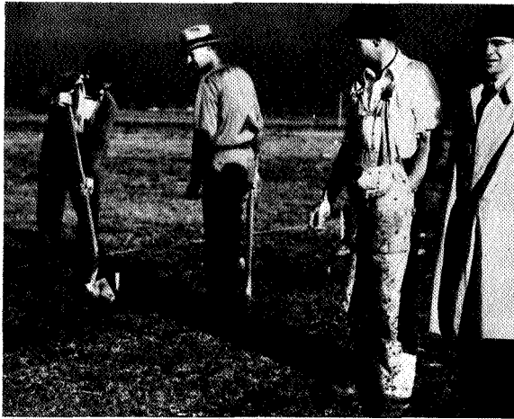
Russell Robinson (right) supervising the first excavation for Ames laboratory Dec. 20, 1939.
