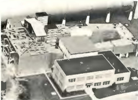
(A) AERIAL VIEW OF ICING TUNNEL
