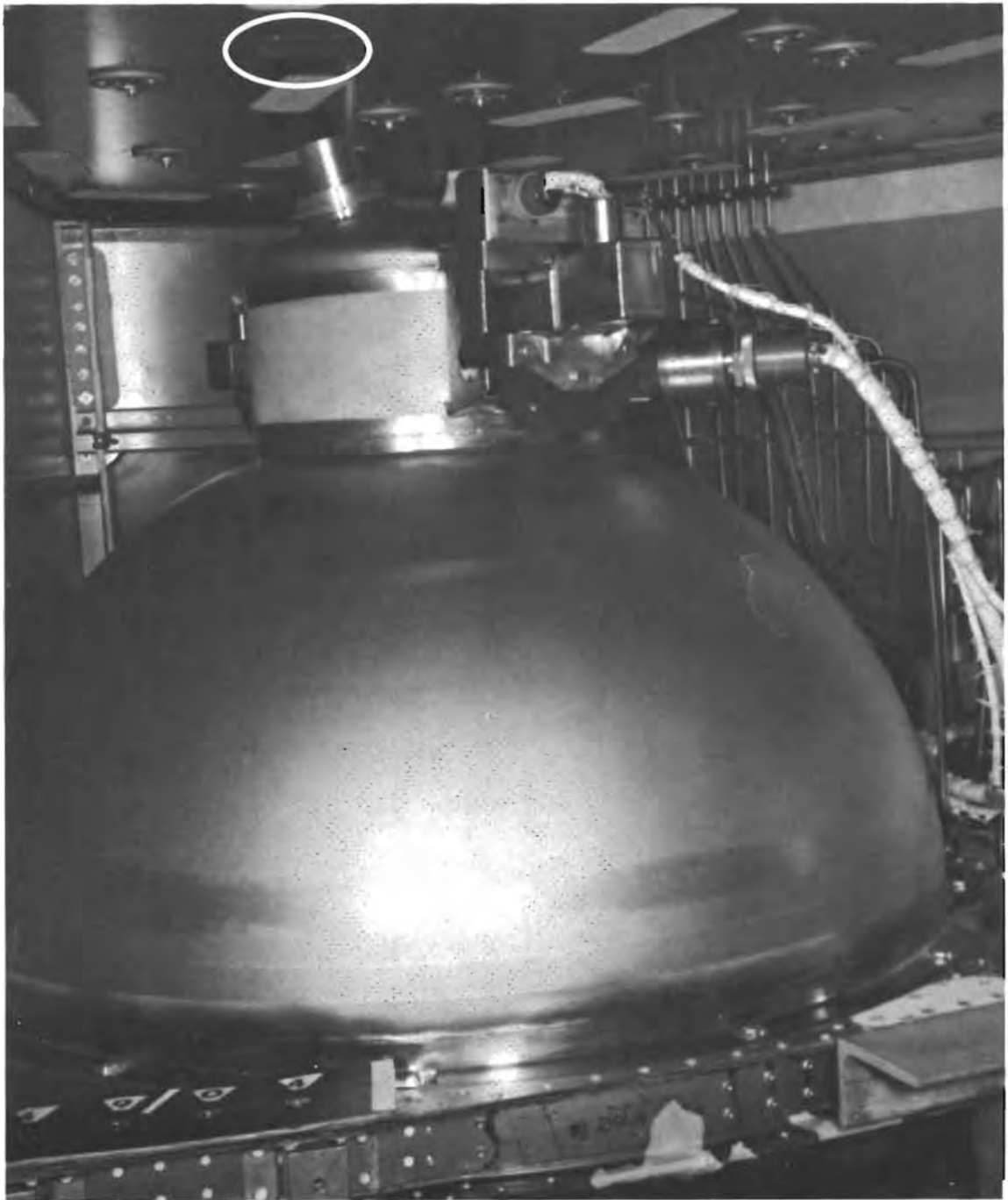
Figure C4-54.- Replacement oxygen shelf installed in Service Module 106. Note repairs to fuel cell snelf over oxygen tank no. 2.
