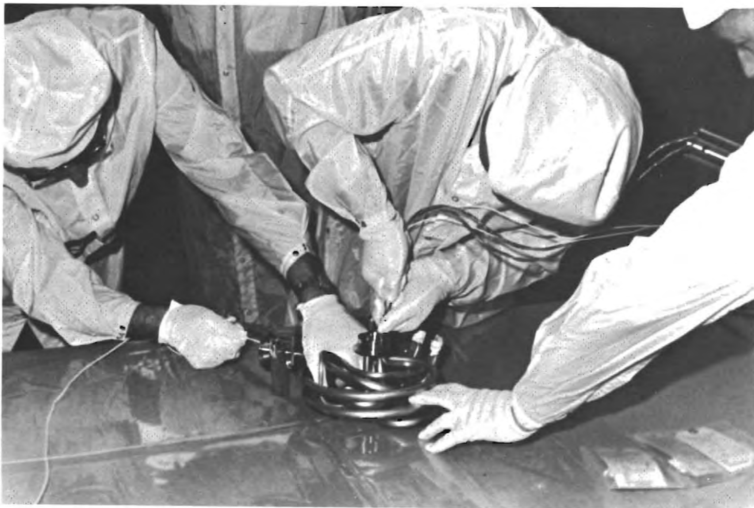
Figure C4-18.- View showing the feeding and pulling used to install wires.
