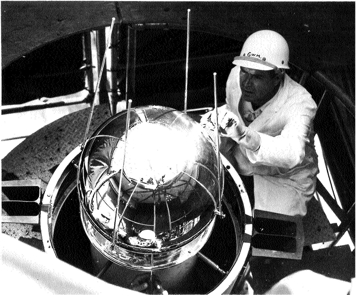
Sketch and photograph of the first of the “operational” twenty-inch Vanguard satellites. It was launched by TV-5, 28 April 1958, but failed to achieve orbit because the third stage did not fire.
