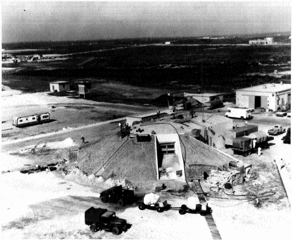
Blockhouse used by Project Vanguard at Cape Canaveral. The horizon window overlooks the launch pad.
