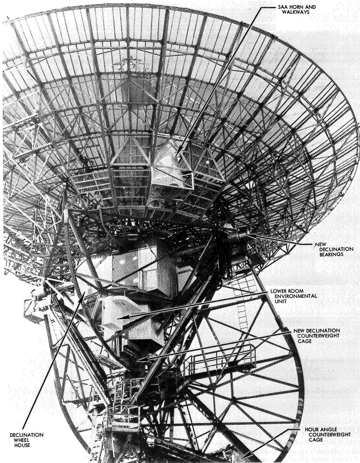
Fig. 77. Antenna structural modifications
