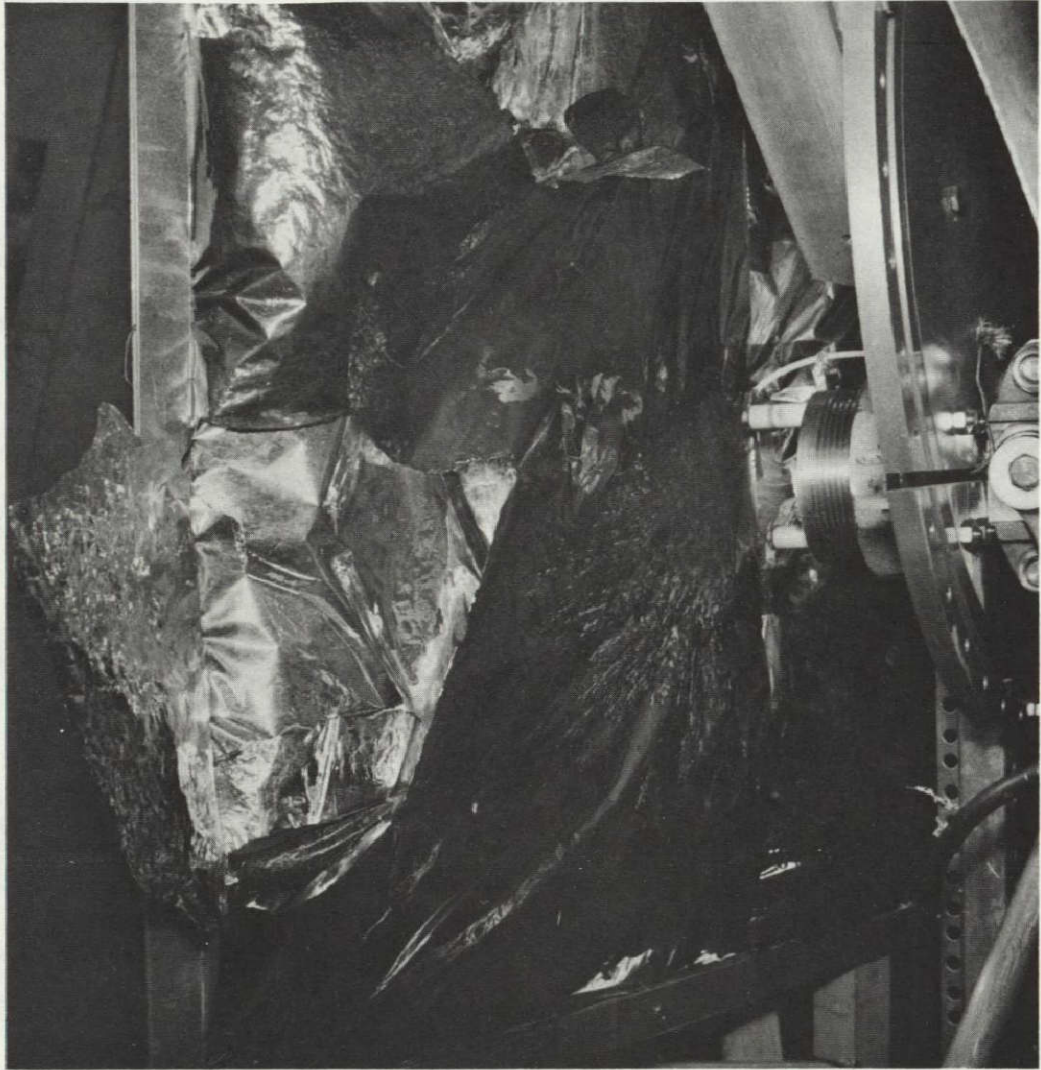
Figure B. 52-2.- Tearing of insulation by 1000 °F stream of oxygen. No burning observed.
