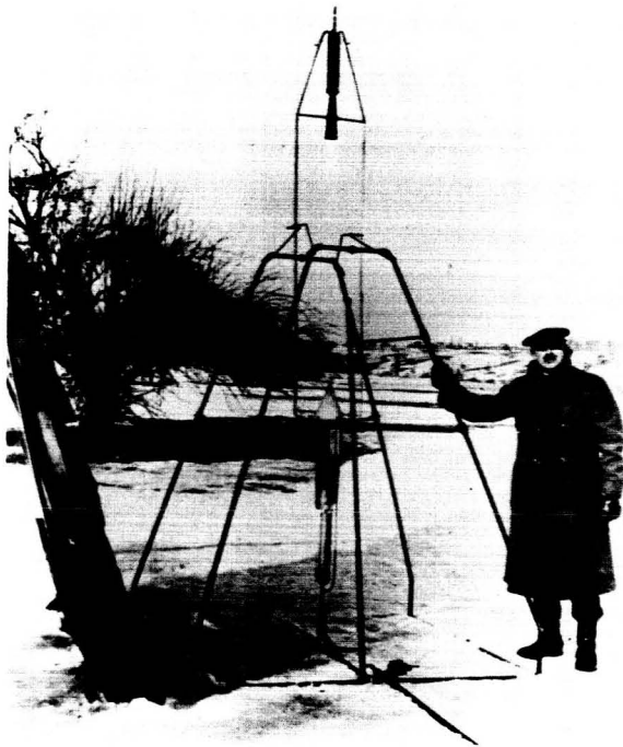
FIGURE 2.—World's first liquid-fuel rocket with its designer, Dr. R. Goddard.
