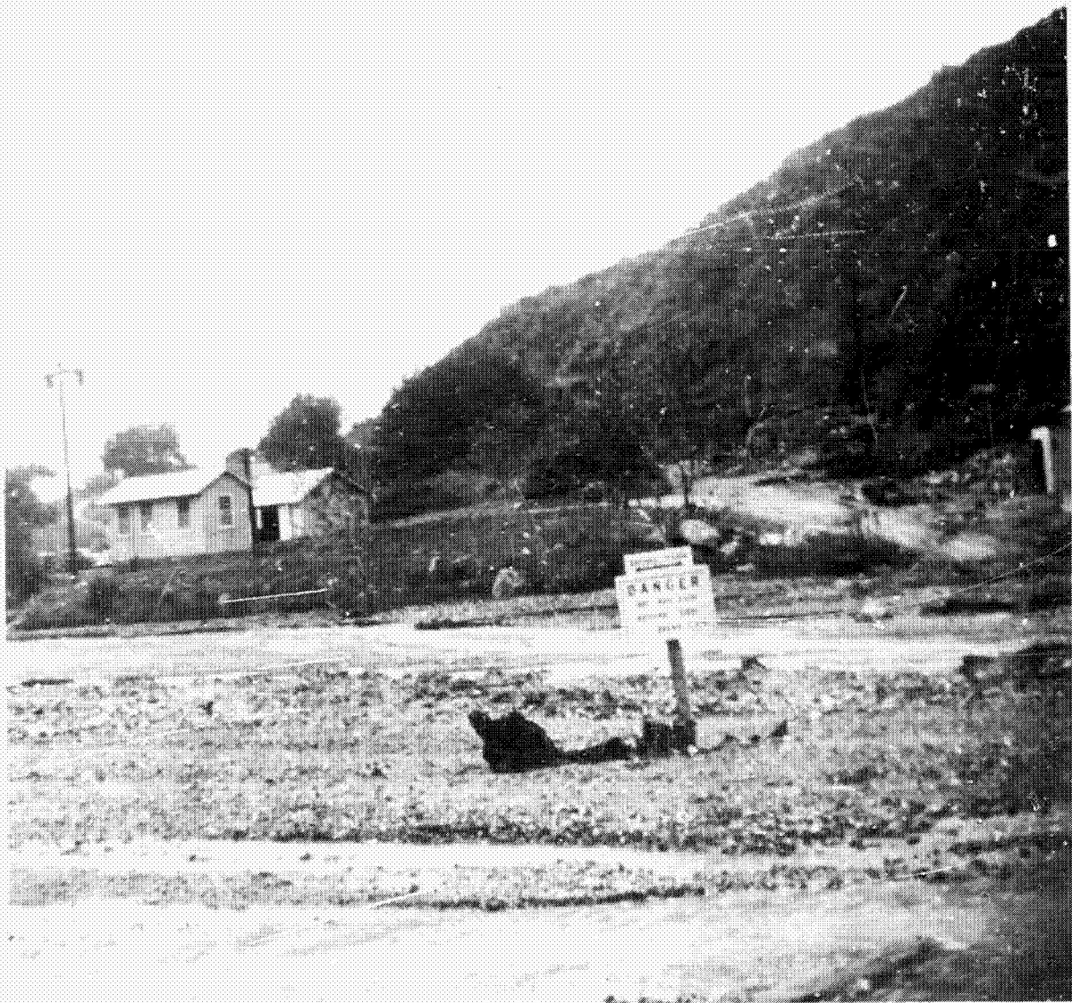
Figure 2: Caltech (JPL) Rocket Research Facility on the Arroyo Seco, fall of 1940. Test pits appear at the far right against the hillside .
