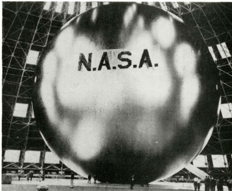
Figure 1.- Fully inflated 41.15-meters-diameter Echo II.
