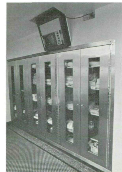
Stainless steel double pass cabinets permit replenishment of supplies through back doors located in the entrance hall.
