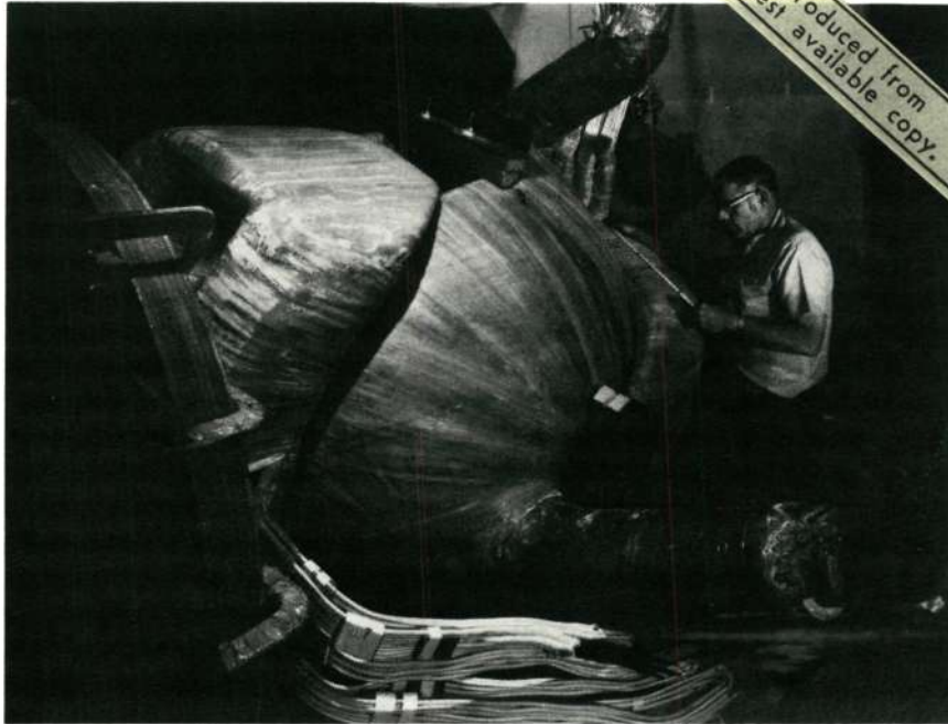
FIGURE 4.66 Photograph of the 2X II pulsed magnet set prior to construction of the external glass and epoxy reinforcement. The completed structure, which contains approximately seven tons of plastic reinforced with glass cloth, is the latest and largest experimental pulsed magnet to be built using techniques that were pioneered at the Lawrence Livermore Laboratory and that are now commonplace in industrial application. [Courtesy Lawrence Livermore Laboratory.]
