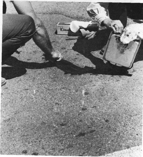
FIGURE 2a MIXING AND APPLYING EXPERIMENTAL QUANTITIES OF THERMOPLASTIC MATERIAL
