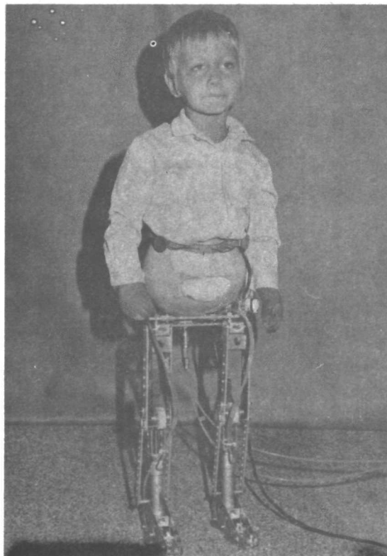
Figure 11. Hydraulic version of prosthesis.
