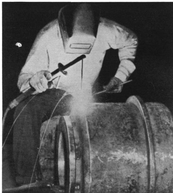
FIGURE 20.—Shielded metal-arc welding of a Hastelloy inlet cooling sleeve.
