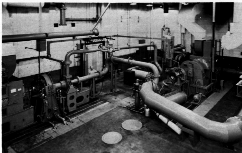
FIGURE 28.—A test facility at Lewis Research Center on which high-speed evaluations of pump inducers and impellers are made through stroboscopic techniques, which appear to slow down the action of the events that occur.
