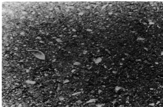
Figure 6—Surface Texture of Fullerton Glasphalt Road after One Year of Service
