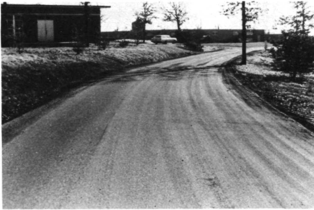
Figure 3—Rolla Glasphalt Road after 30 Months of Service
