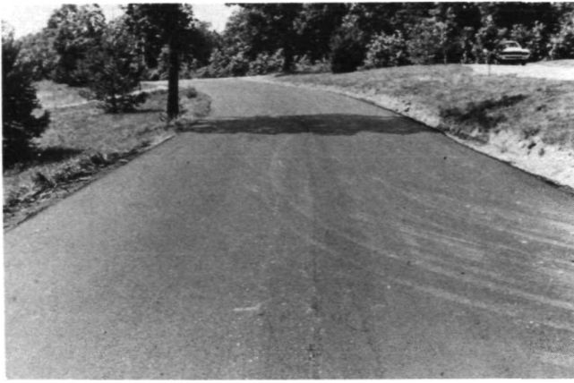
Figure 1—Rolla Glasphalt Road Immediately After Placement
