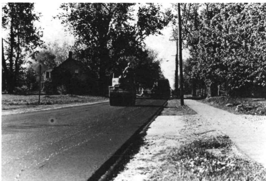
Figure 9—Rolling of South Burlington Glasphalt Road
