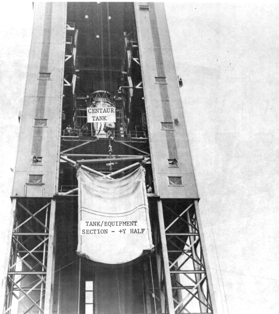
FIGURE C-4 SHROUD INSTALLATION - TANK/EQUIPMENT SECTION
