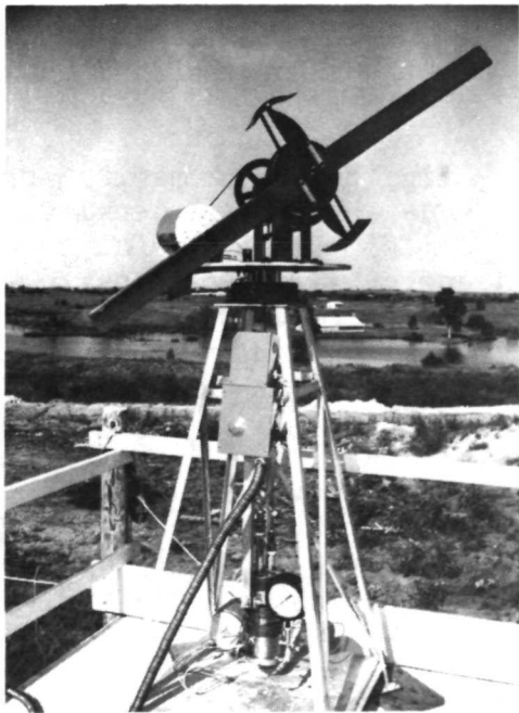
Figure 11. Close-up view of the experimental prototype wind energy storage system.
