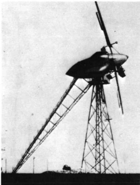
30 m \phi . 100 KW DC RUSSIAN WIND-TURBINE, YALTA, BLACK SEA, 1931.
