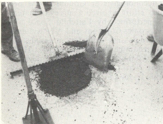
Thermoplastic material is being adapted for bridge-surface coating and road repair.
