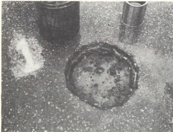
The hole was filled with thermoplastic material that was originally developed for binding solid fuels used in rockets.
