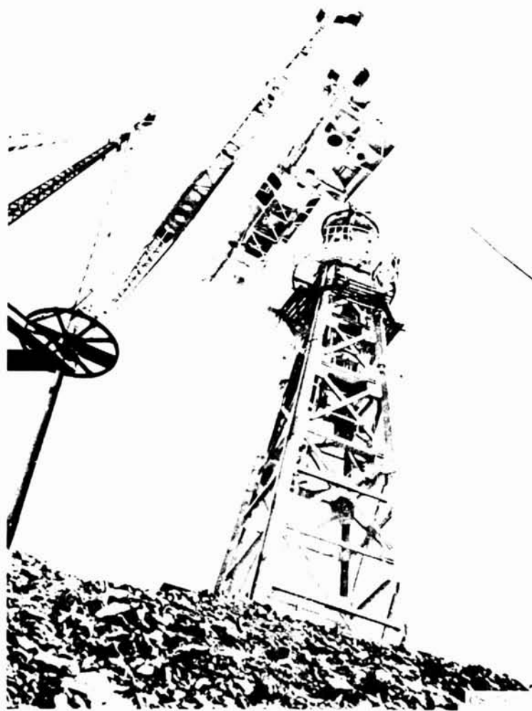
(b) A view showing the generator housing platform being lifted onto the top of the tower.
