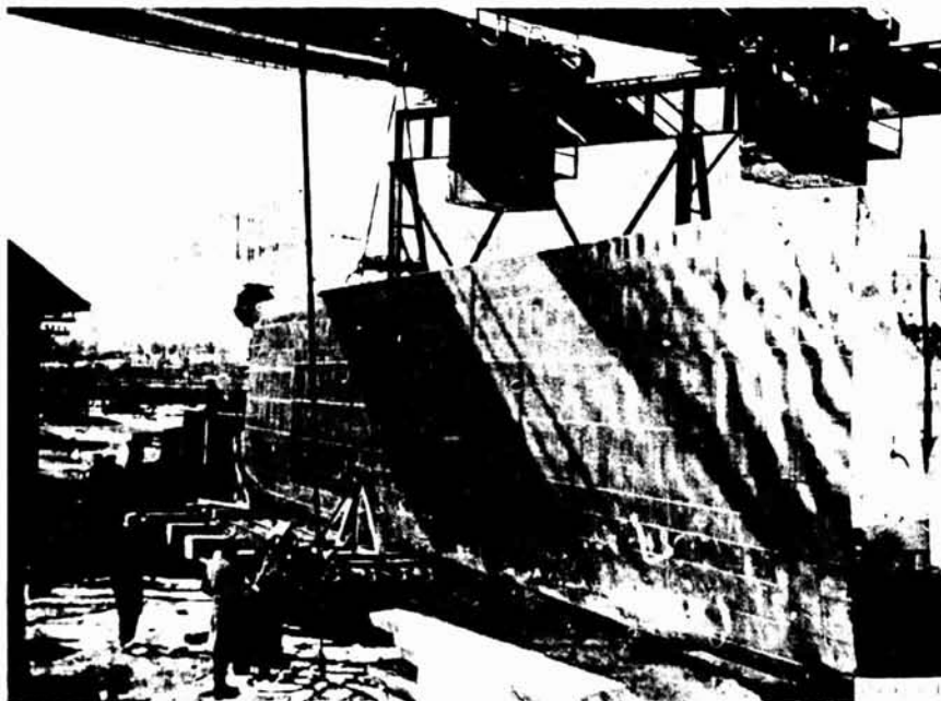
(d) A view of one of the rotor blades at the base of the tower being readied for hoisting into place at the top.
