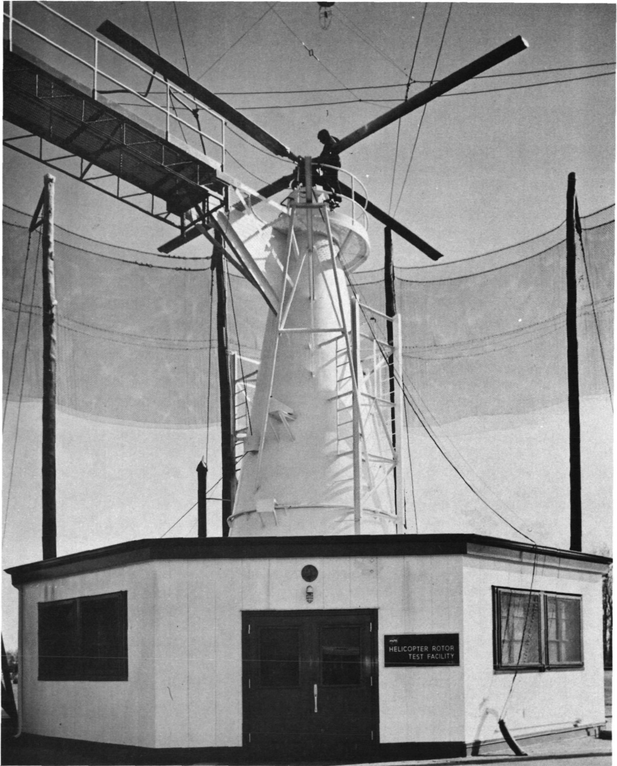
Figure 1. NASA Langley Research Center Helicopter Rotor Test Facility
