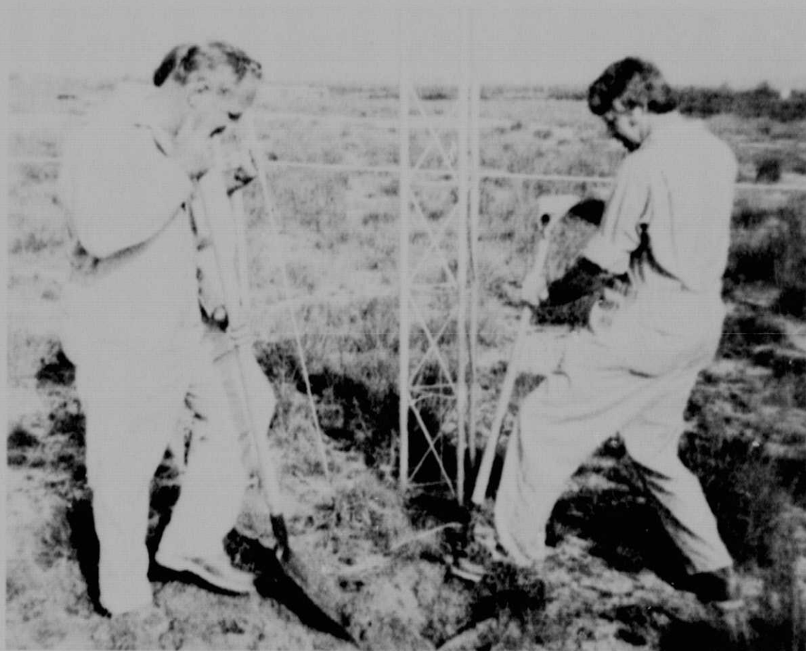
Fig.6-8 - Erection of Calibration Target Tower
