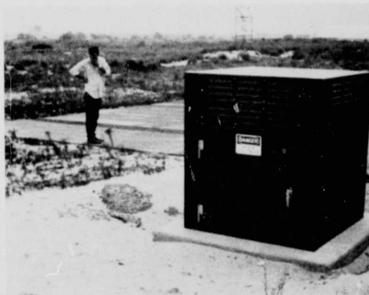
Fig. 6-2 - Pad and Power Transformer for the No. 1 SLDS Unit
