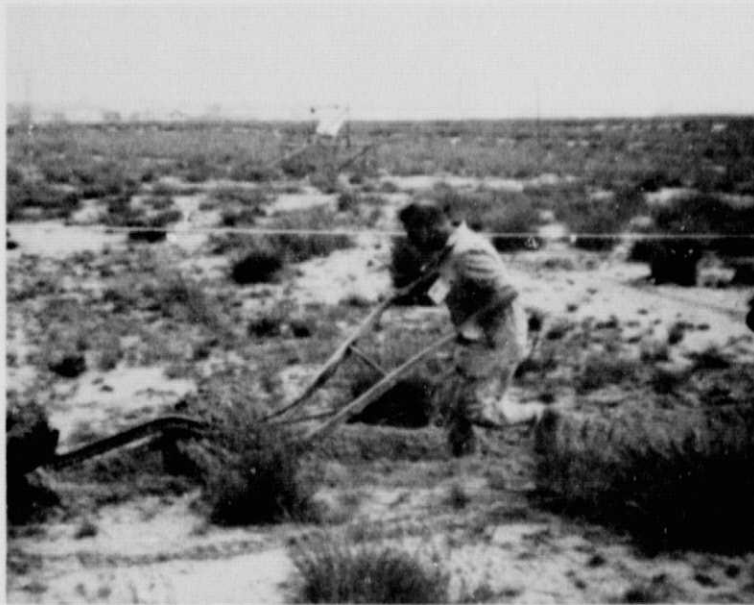
Fig. 6-7 - Modern Ditching Technique for Cable Interfacing Between Vans 1 and 2
