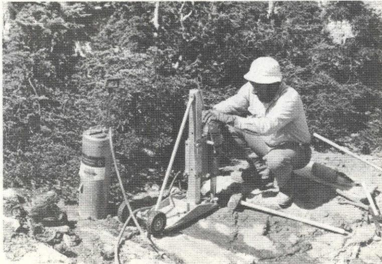
Figure 6. Drill used to drill hole in rock for tiltmeter
