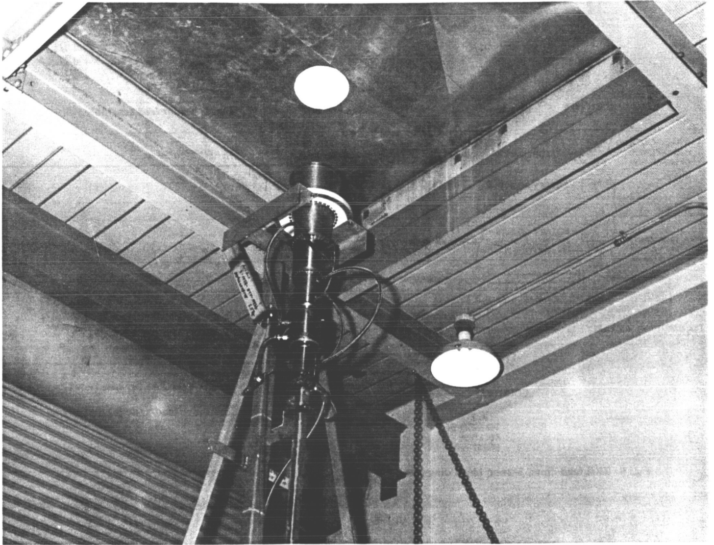
Fig. 7. Radar feed assembly power tests
