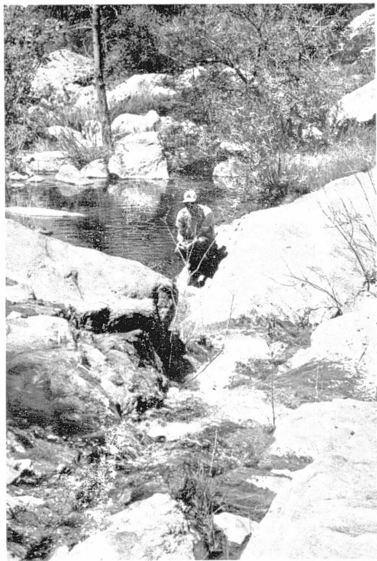
Fig.18 - Exposure of fault surface along San Diego River fault zone at point D, Fig. 14.
