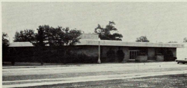
Figure 3.— One-story masonry building. Point of reference: front.
