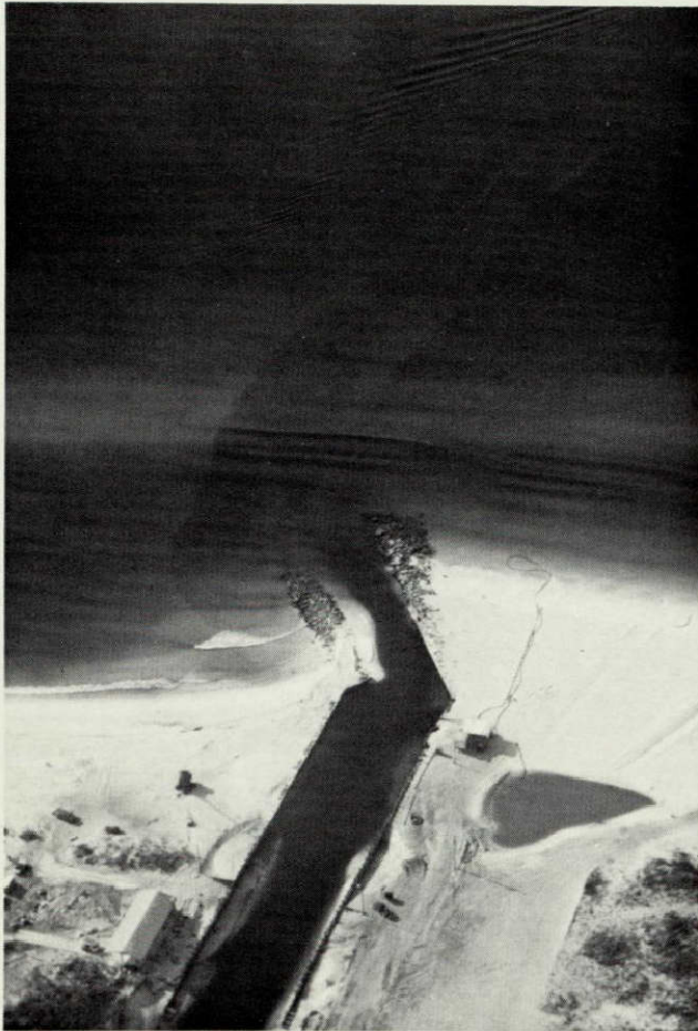
Figure 5.— Shoal harbor entrance: Example of ineffective navigation structure.
