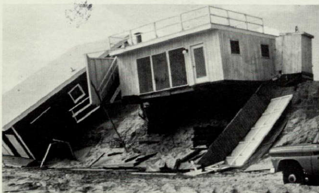
Figure 6.— Coastal damage: result of sediment movement.
