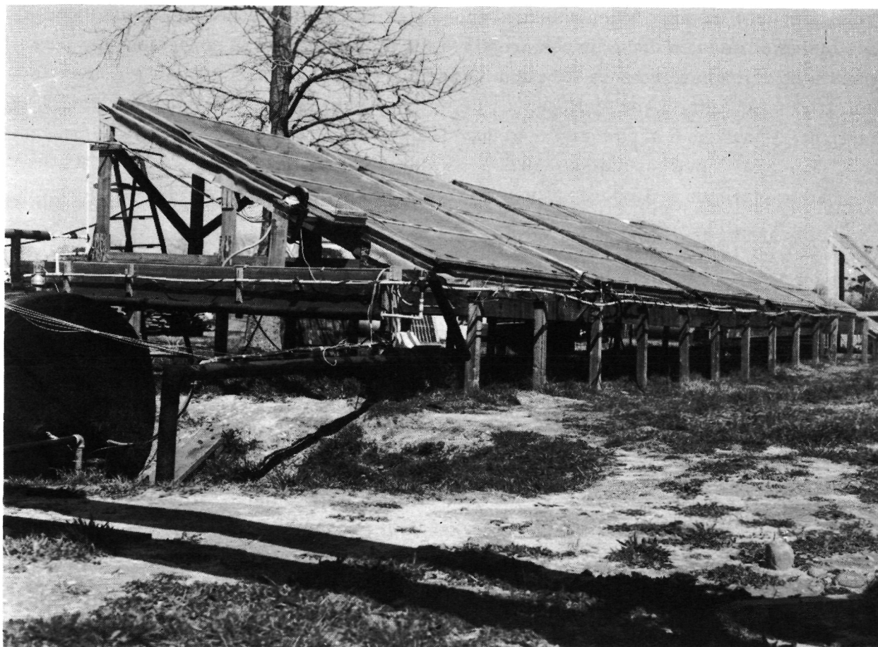
Figure 1.- Photograph of solar collector array.
